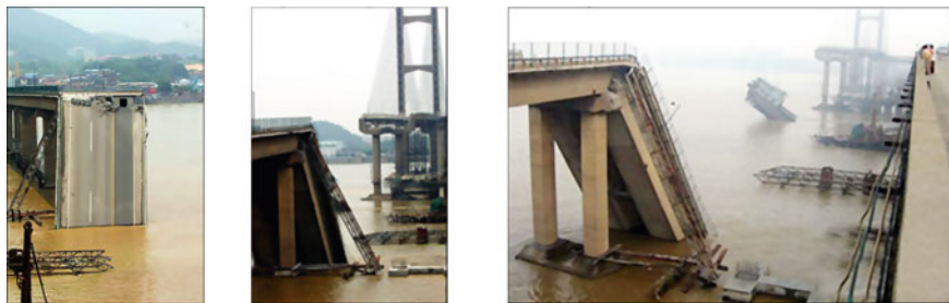
Fig. 1 Accidents of ship on RC piers of Jiujiang Bridge in China [9]
