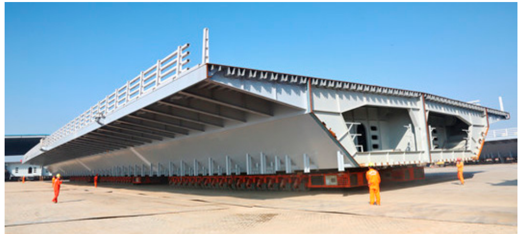
Figure 1. Steel box girder.
